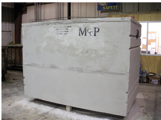
Prepped grease trap structure ready for lining.
