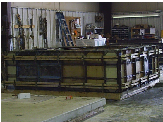
Climate controlled precasting area.
